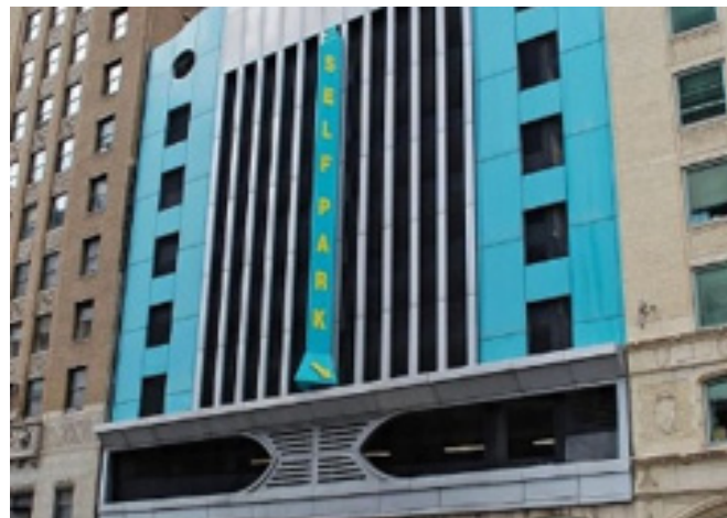
Foto 9. Self Park Garage (1986), Chicago, Illinois [23]
